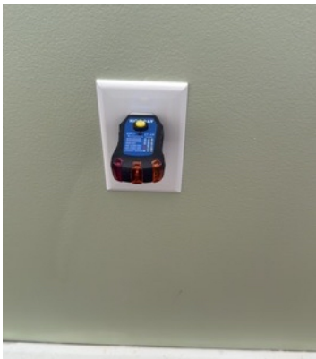
Below Living Room Windows
